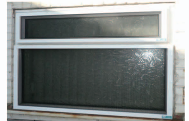
After Intruder Shield Installation
