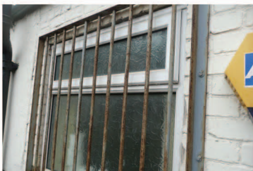
Before Intruder Shield Installation
